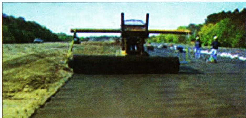
TemPark is a roll out surface that is water-permeable, as well as mold-, mildew- and UV (ultraviolet)-resistant.
